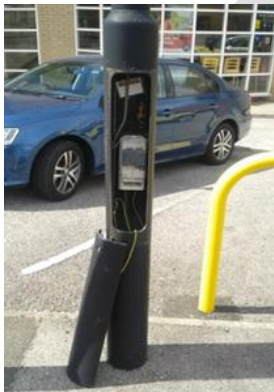
Lighting Column access cover Removed exposing cables
